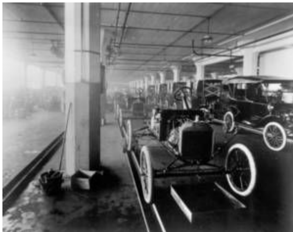
Model T engines on assembly line at Ford Motor Company plant, Highland Park, Michigan, about 1914
